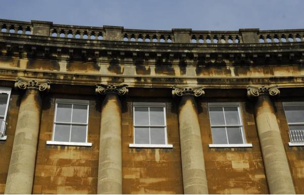
Detail of weathering pattern to elevation
