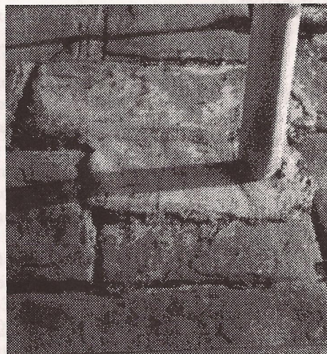
Above, a repair outside No 1 - three uneven pieces of paving have been laid to replace one.
