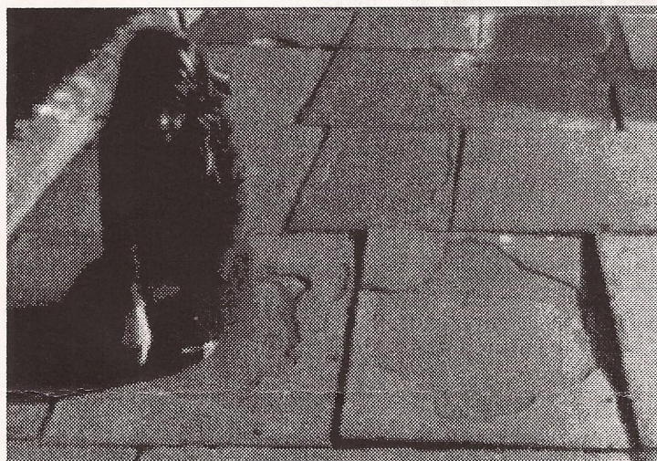
Above, a repair outside No 1 - three uneven pieces of paving have been laid to replace one.
