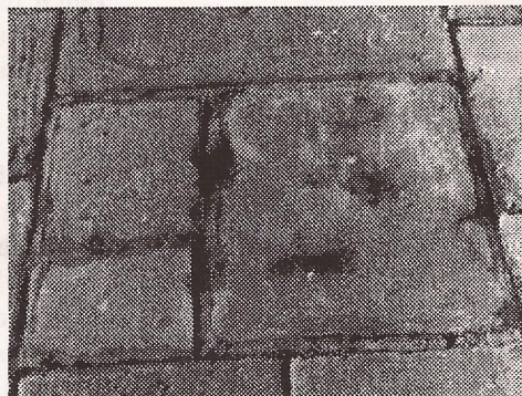
Above, a repair outside No 1 - three uneven pieces of paving have been laid to replace one.
